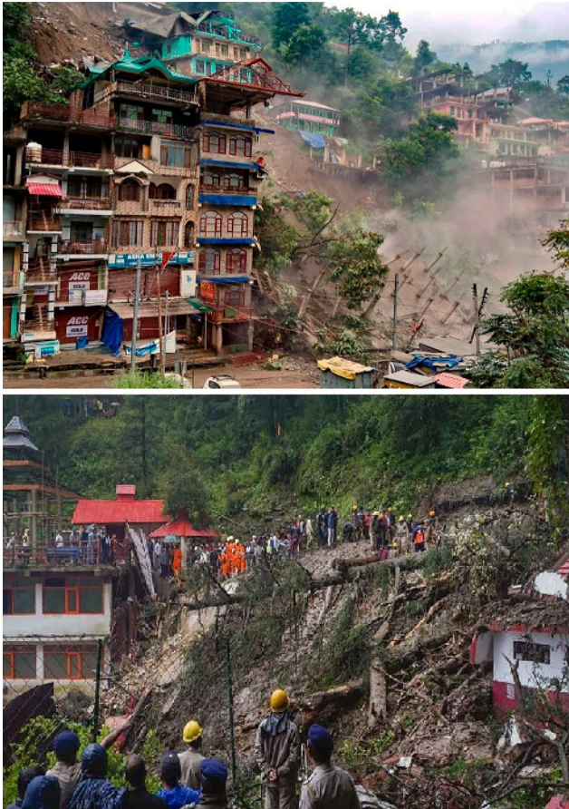
Figure 1: Floods and landslides in Solan district of Himachal Pradesh.
